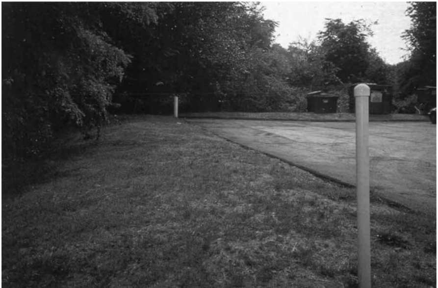
Photo 5.3c Final view of the area where the trench is now dispersing the effluent from a SBR treatment system. Note that one end of the “L” shaped trench is at the white observation pipe and the other end is next to the dumpster.
