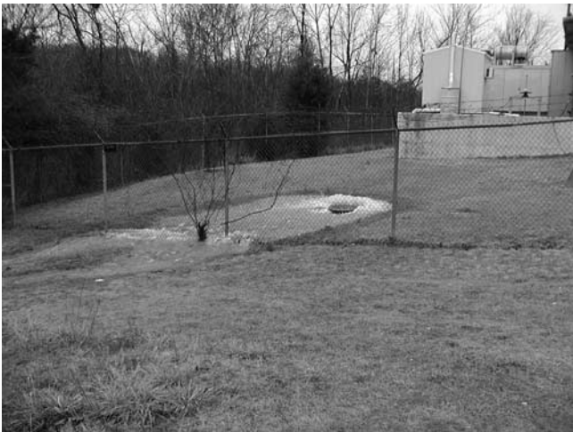
Photo 2.2 City sewer system facing problems due to I & I – Note the over flow of raw wastewater from the manhole and the backup power generator in the background.
