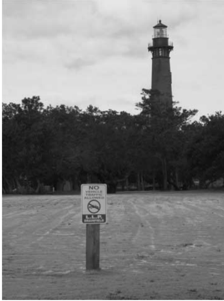
Photo 5.8a Effluent dispersal area with a sign to restrict any vehicular traffic within the area.
