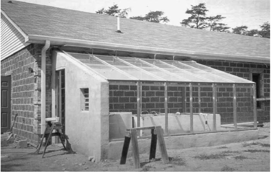
Photo 5.10a A wetland treatment system installed within a greenhouse for dispersal of effluent directly into atmosphere in form of humidity. This system serves a community center. Note the picture is taken just before the system went online.
