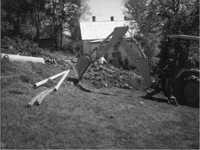
Photo 5.1a Installation of a small (10-ft long and 1-ft wide) trench on a slope. Note that the backhoe is digging in the trench just by scratching the ground surface.
