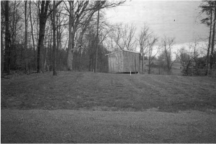
Figure 5.4b Drip dispersal system area a few months after installation. Note that the grass is established and under the grass cover, effluent from an advanced onsite system is dispersed using drip lines.
