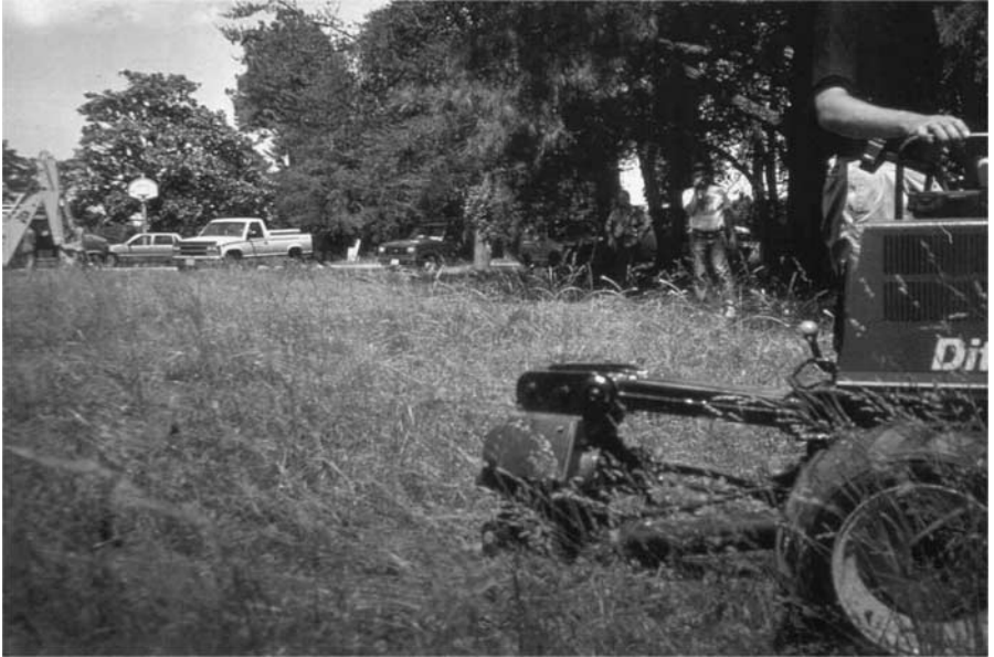
Photo 5.5a Drip system for effluent dispersal installed in open area using a vibratory plow. Source: Photo courtesy of Mr. Robert Mayer of American Manufacturing, Inc., Manassas, VA.
