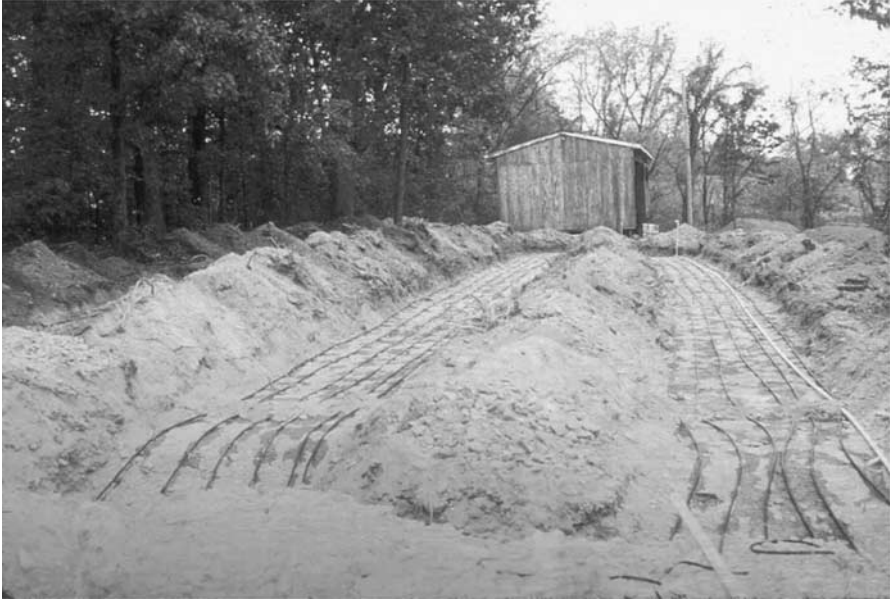
Photo 5.4a Drip dispersal system for an individual home. Note that the drip tubing is installed in five feet wide trenches. Trenches are open and the system is being tested before covering the trenches.
