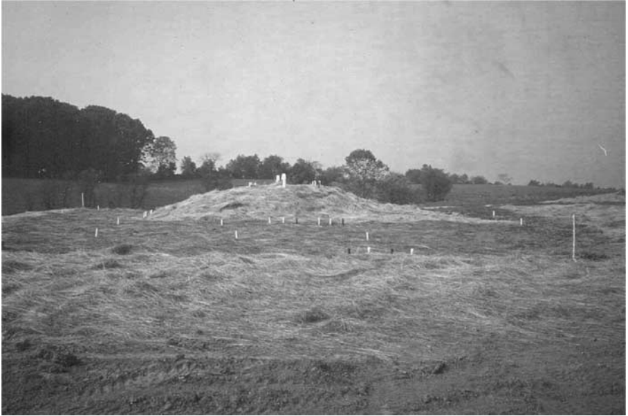
Photo 5.7a A filter bed system for dispersal of effluent from an advanced onsite wastewater treatment technology that serves a single family home. Note this picture was taken a few days after the installation was completed.
