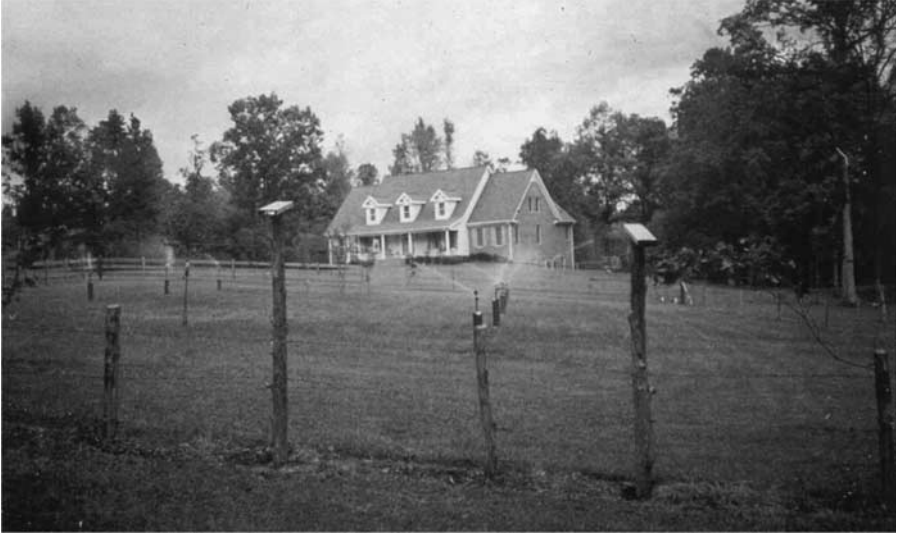
Photo 5.6a Spray irrigation system installed in the front yard used for dispersal of effluent from an advanced onsite wastewater treatment technology that serves a single family home.
