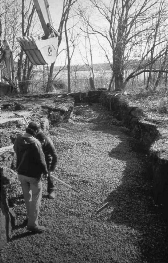
Photo 5.3a A 5-ft wide and about 100-ft long trench that was dug down to about 10-ft depth to the sand layer and filled up with gravel. The “L” shaped trench is used to disperse about 5,000 gallons per day effluent from an advanced onsite treatment system that serves a service station. Photo courtesy of Mr. Daniel Pavon of Aquarobic International, Winchester, VA.
