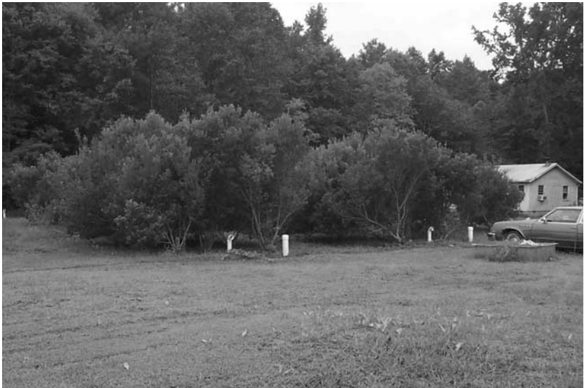
Photo 5.9b Evapo-transpiration beds about four years after the installation. Note the plant growth within the beds.
