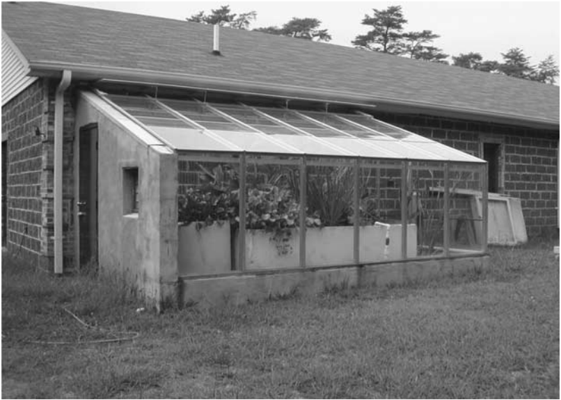
Photo 5.10b The wetland system within the greenhouse a few years after the system went online. The final effluent from this treatment system is disinfected using Ultra-violet light disinfection system and the disinfected effluent is reused for flushing toilets inside the community center.
