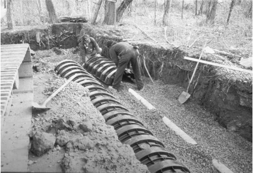
Photo 5.3b Chambers were used to cover the four inch perforated pipes placed in the trench. Photo courtesy of Mr. Daniel Pavon of Aquarobic International, Winchester, VA.
