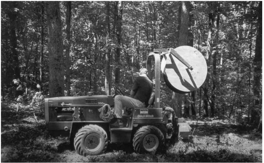
Photo 5.5b Drip system for effluent dispersal installed in wooded area using a vibratory plow.
