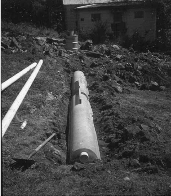
Photo 5.1c Side view of the small and shallow trench before covering the trench with soil material removed from the area.
