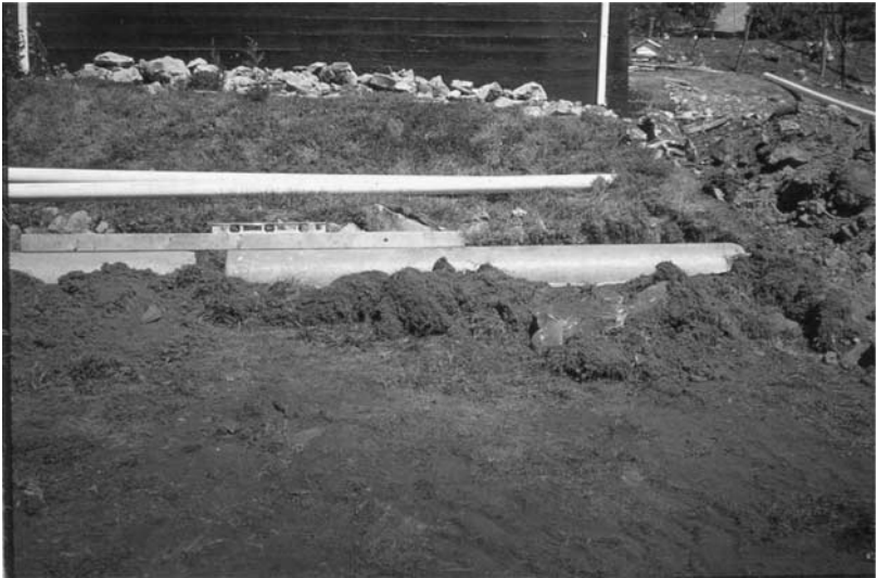
Photo 5.1b Close view of the small and shallow trench. Notice the fiberglass cover placed on typical four inch perforated drain pipe placed in the trench. There is no gravel used in this trench.
