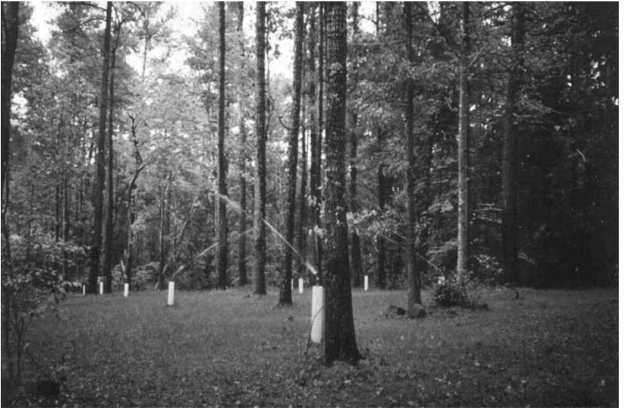
Photo 5.6b Spray irrigation system installed in wooded area, back yard of a house, used for dispersal of effluent from an advanced onsite wastewater treatment technology that serves a single family home.
