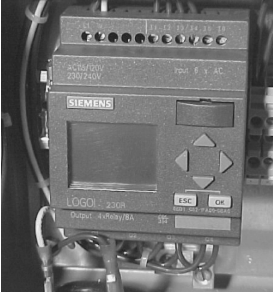
Photo 3.2 Programmable logic controller
