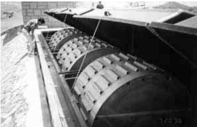
Photo 4.1 Rotating biological contactor.
